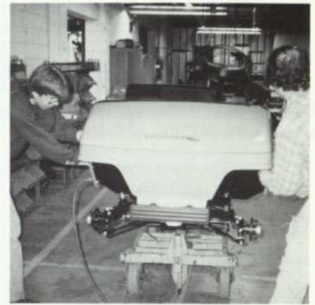
Vehicle controls are being installed here.
