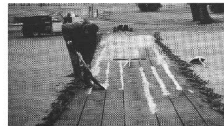
Backfilling trenches with sand.
