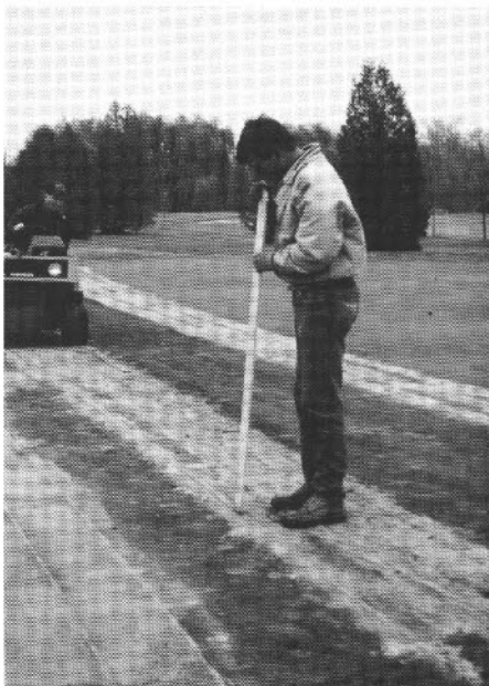
Turf students compacting trenches with sand.
