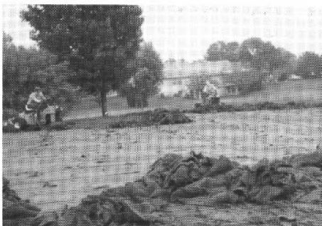
Bull-dozing sod in piles
