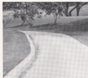
Curbed cart path.
