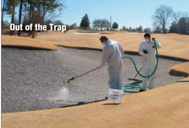
Better Billy Bunker worked with Dow to formulate a sprayable polymer that binds the gravel together, eliminating the need for a liner.
