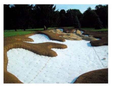
Milliken & Co. offers the SandMat Bunker Liner, available in three versions to meet specific needs of golf courses around the world. SandMat provides architects with design flexibility, builders with high-quality product delivered in the widest rolls for installation ease and lower cost, and golf course superintendents with bunkers that stay more consistent and are better playing with lower maintenance costs. The best thing about SandMat is its rain-event performance, according to Milliken & Co.
