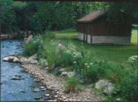
Streambank rocks and plantings can prevent erosion, stop unnecessary mowing and provide aesthetic appeal.
