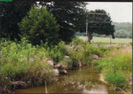
Rootwads stabilize the streambank while letting riparian shrubs to establish.
