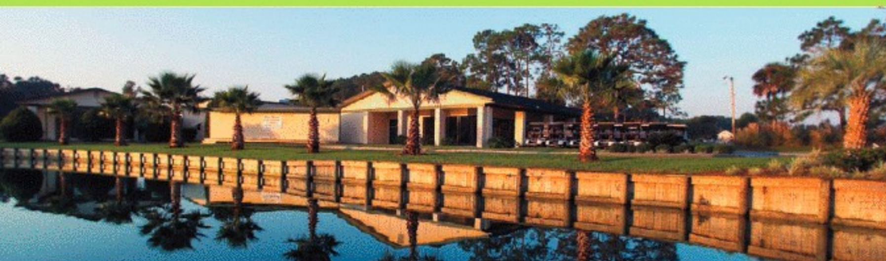
Above, the proposed Selva Marina clubhouse features smaller, more purposeful rooms, a coffee bar and WiFi connectivity. The current clubhouse (below) fails to incorporate enough useful outdoor spaces to meet the needs of the Atlantic Beach community.
