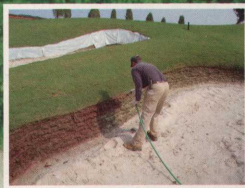
Sod-sided bunker face being stabilized and tinted.
