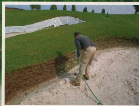
Sod-sided bunker face being stabilized and tinted.
