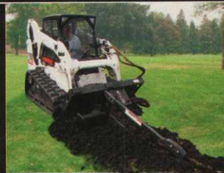
Track loader trenching irrigation line
