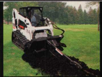
Track loader trenching irrigation line
