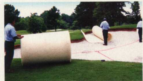
Sandtrapper for bunker renovation
