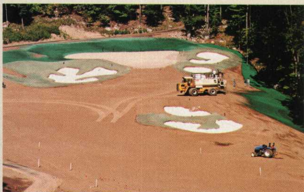
A test showed that an application of the fiber matrix material reduced erosion by almost 100 percent compared to bare, untreated soil.
