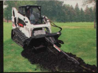
Track loader trenching irrigation line
