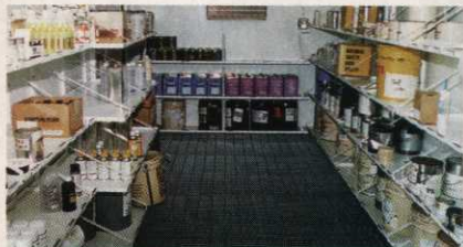
Building equipped with shelving for storage of bottles, cans, buckets, bags, and boxes of chemicals and other materials.
