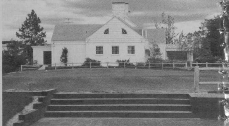
Top, if steps are not of the right design proportions, golfers will not use them and a worn area will develop to either side. Bottom, this is another view of the tee at Faragote from the practice green.
