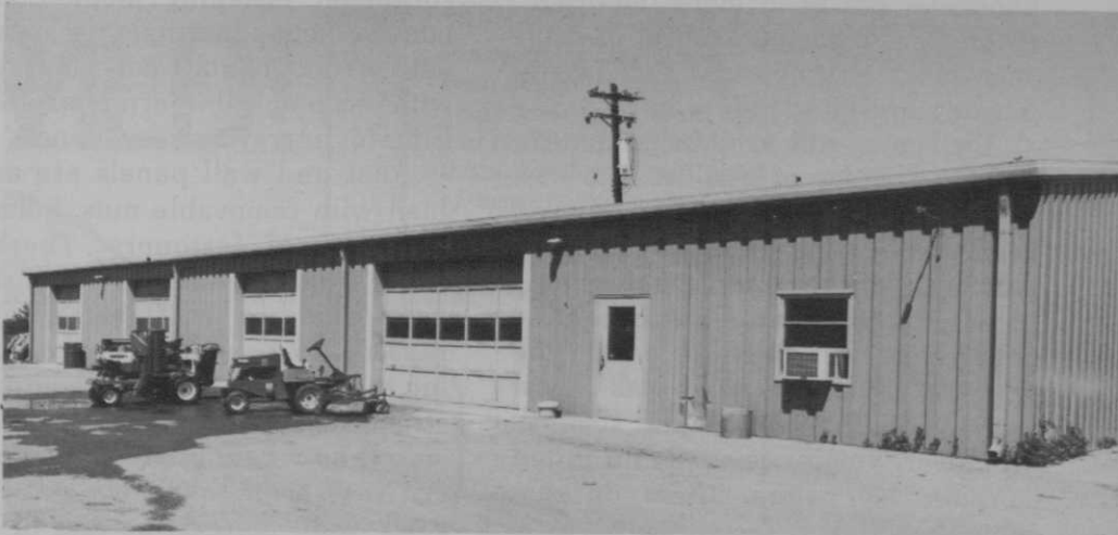
Interior and exterior of maintenance building at Middletown's Weatherwax Golf Course in Ohio. Note how high ceiling permits step-up storage above office and stockroom.
