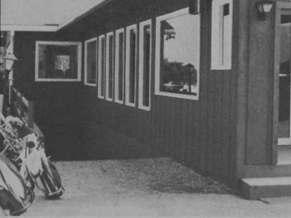
LEFT: Ramp next to pro shop leads to basement of clubhouse, where golf cars are stored and maintained.
