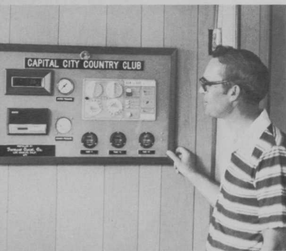
Some 550 sprinklers on the course at Capital City CC are controlled from a master panel in Superintendent Roy Conard's office.
