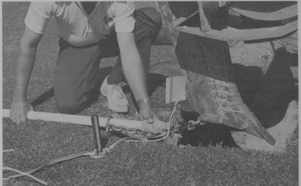
Pipe is attached to vibratory plow blade with pulling grip.
