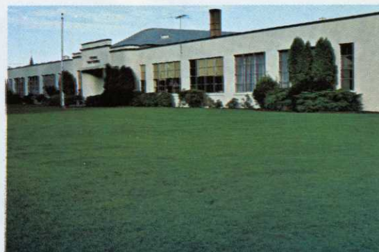
School grounds in St. Paul, Oregon gets plenty of traffic but still looks great.
