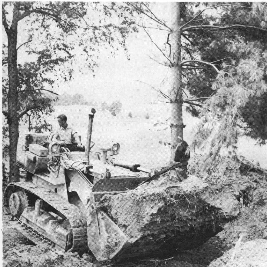
Taking advantage of nature: During construction of the Bellville Project, repositioning of existing trees helped give the course an established look. At the same time, the owners acquired a substantial savings over the cost of replacement stock. Several hundred white pines were transplanted.
