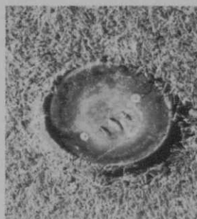
Reject concrete pipe was used on some holes to carry water under the fairways from canyons above so the course would not have water problems on the fairways.
