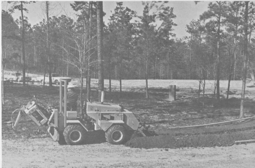
Davis Fleetline 70+4 with P-80 Line-Layer pulls in pipe for automatic irrigation system on hallowed turf at St. Andrews Golf Course in England, where game of golf was invented.
