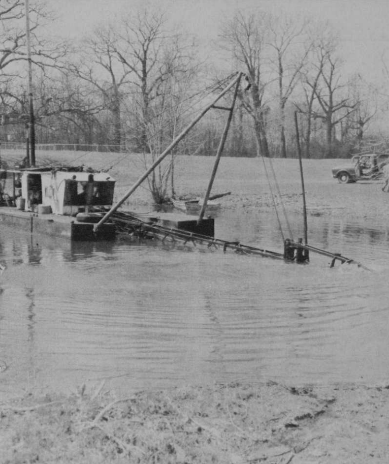
The portable dredge lies in the 1½-acre reservoir (top left). Cutting in a semi-circle, the dredge took out 2,600 cubic yards of silt and weeds working, in as little as two feet of water (top center). Over 1,500 feet of pipe was used to carry the discharge material (top right).
