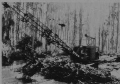
Useless swampland (above, left) was dug out and cleared with heavy machinery (left), then dredged (above) to form an attractive and functional water hazard at the Innisbrook CC, Tarpon Springs, Fla.
