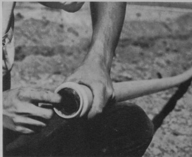
The bell is an integral part of the PVC plastic Ring-Tite pipe. Here rubber ring is being inserted into groove in bell. Ring helps speed assembly, absorbs pipe expansion and contraction, triple seals joint against leaks.
