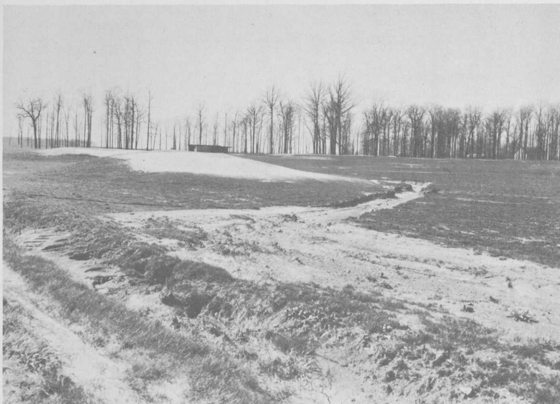
Erosion of newly seeded golf course can be seen around sand trap, and in filling of road ditch.
