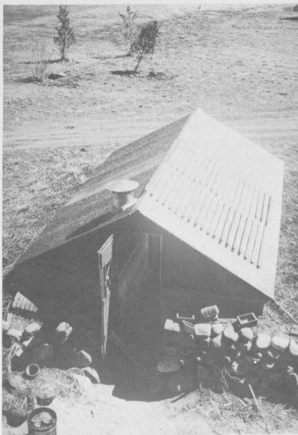
One of last year's off-season projects at Boulder CC, was building this greenhouse. The snow fence on the roof is to shade tender plants.
