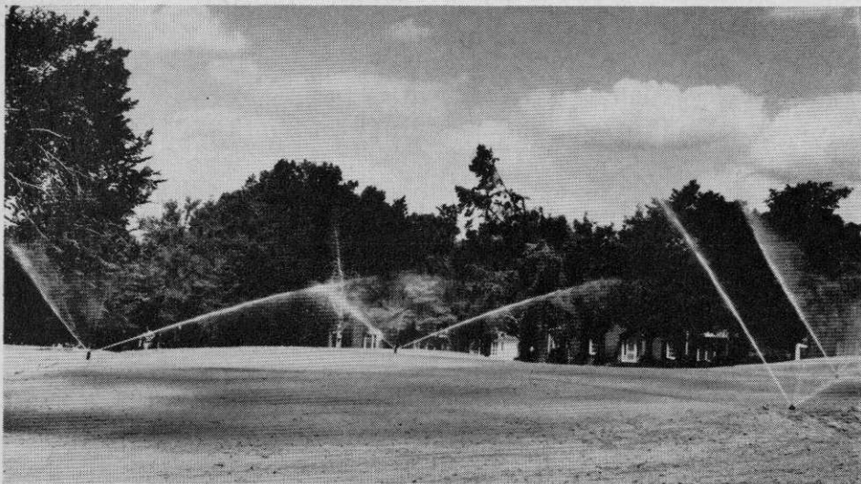
Green's sprinklers are started after mulch and seed are spread by the hydro-seeder.
