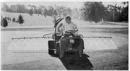
**USE IT AS A SPRAY RIG** with boom for spraying greens, without boom for large areas, or with hand sprayer for trees and shrubs. Entire spray rig lifts off easily when not in use.
