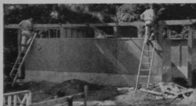
Installing main roof beam
