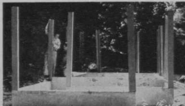
Corner posts being set in position
