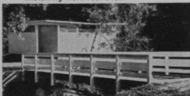
Completed and Painted Comfort Station
