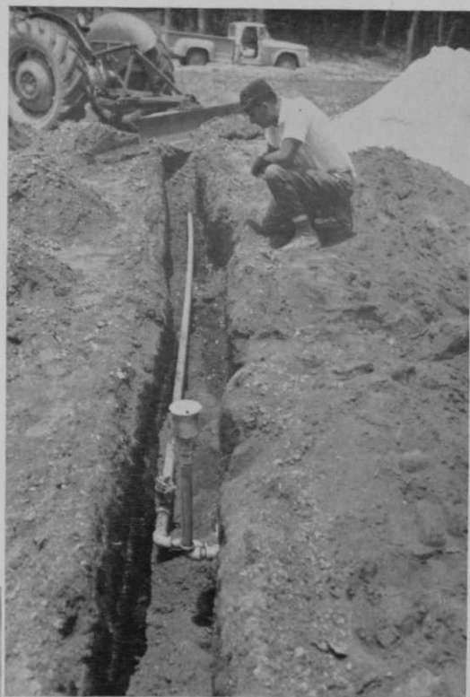
The watering system is made up of five pop-up sprinklers which ring each of the greens.
