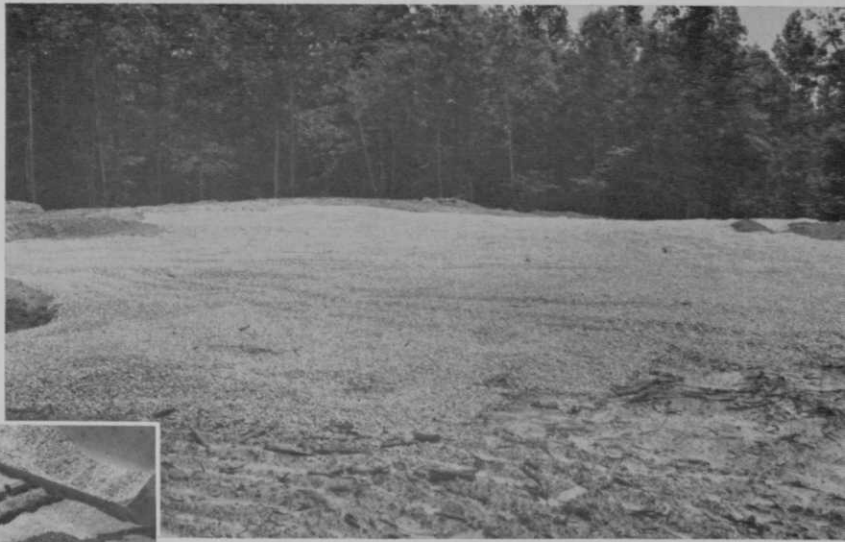
This view shows the 4" of \frac{3}{4} " stone which has been spread over a rough grade to form new golf green at MacGregor Downs.
