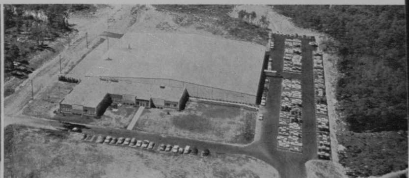
Aerial View of New Home of Miller Golf Company
