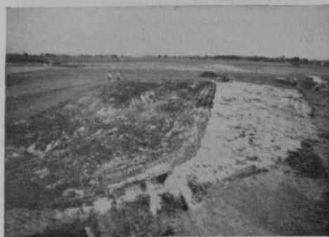
After topsoil has been laid, additional Turface is worked in by discing.
