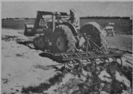
Next, it is mixed. A farm harrow breaks up soil chunks and works Turface in.
