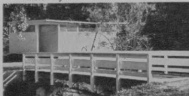
Completed and Painted Comfort Station
