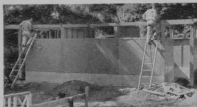
Installing main roof beam
