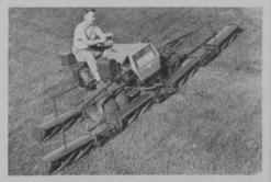
Kohler engines, and three cutting widths, units have heights of cut from one-half to three in. and are changed easily. The smaller model is equipped with either three-reel units to mow an 81-in. swath, or five-reel units for an 11-ft. width of cut. The 18-hp Super Pro may be fitted with either a five or a seven-reel unit. The latter cuts a 154-ft. swath.
