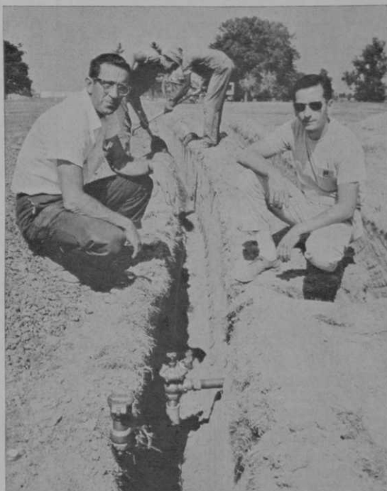
Dick Betterly, left, superintendent for the prominent irrigation specialists, A. J. Miller, Inc. of Royal Oak, Michigan, and Mark Schurman, right, inspect one of the automatic angle valves in the CRESline system.
