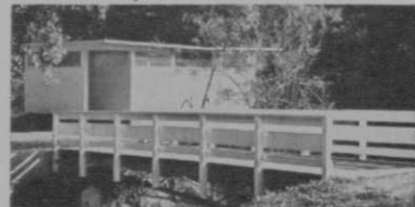
Completed and Painted Comfort Station
