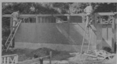
Installing main roof beam
