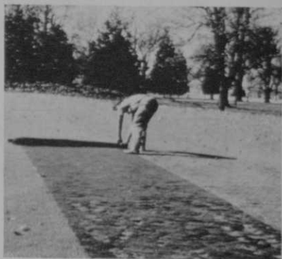
One man easily installs and re-rolls Famcomat. Tests have proven Famcomat can be effectively re-used as many as three times.
