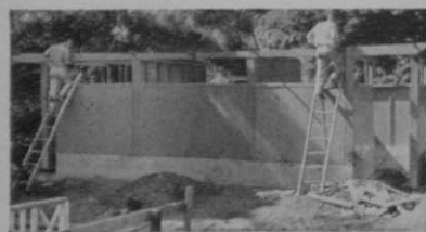
Installing main roof beam
