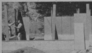
Coded panels being set in place
