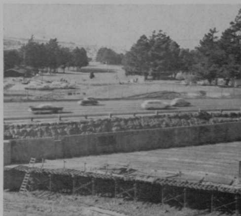
Freeway excavation, which took about a 13-acre slice out of the San Francisco course, goes on in the foreground. Traffic is being temporarily routed over Junipero Serra boulevard.
