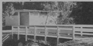
Completed and Painted Comfort Station
