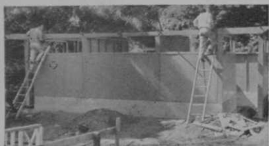
Installing main roof beam
