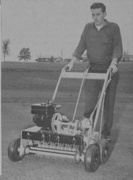
You'll do up to 1/3rd less watering . . . have greener, better-playing greens . . . when you keep your greens well aerated with the Ryan Spikeaire during hot, dry weather. The Spikeaire cuts through the thick, hard crust that forms on the soil surface, making tiny openings that relieve the surface compaction and let water soak directly
