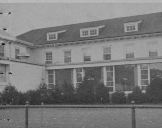
Practice green, just outside Pro shop front door, is located in clubhouse offset. Directly behind it is the main dining room.
