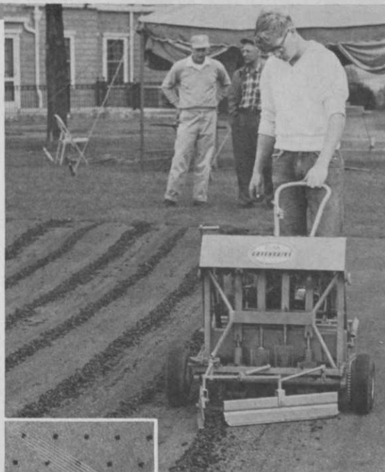
Coring immediately relieves compaction so ball "bites" on green—and rolls true.
