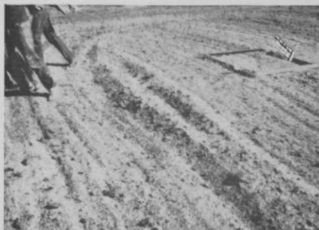
Using a drag, the treated topsoil is levelled before seeding or sodding.
