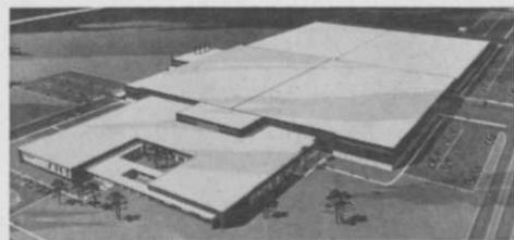
Overall view of the national headquarters of Wilson Sporting Goods Co., River Grove, Ill.
